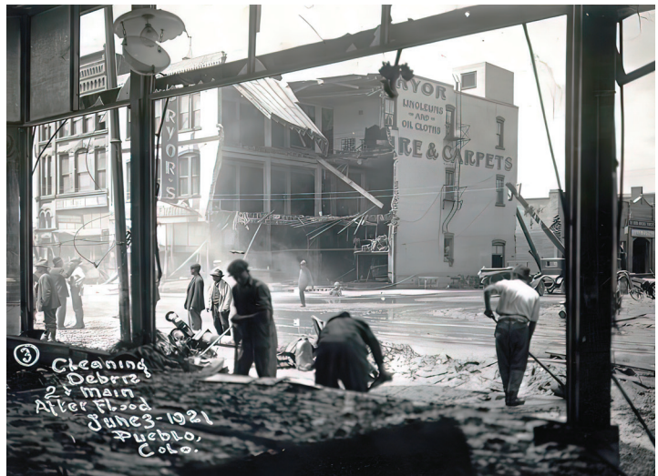
Courtesy Pueblo County Historical Society Pryors Furniture Store, showing the Extent of the Damage to the Building
