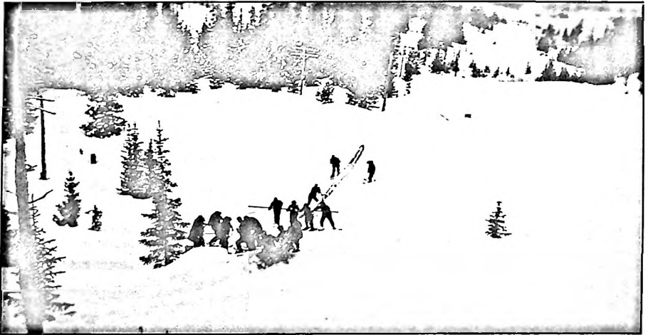
In these photos a crew on snowshoes pulls a replacement pole and installs it on the Shoshone transmission line near Argentine Pass.
