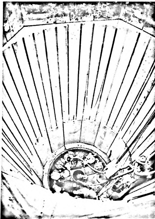
Courtesy Denver Public Library, PSCo collection, WH1367 The prestressed concrete reactor vessel was cut up and removed leaving a large hole
