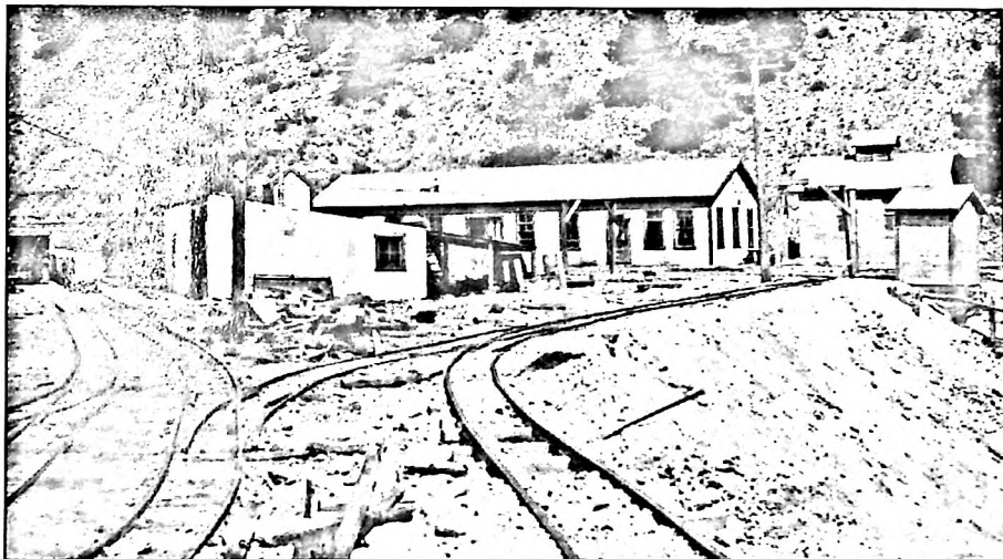
Newhouse-Argo Tunnel, showing powerhouse and trackage, Sept. 30, 1908
