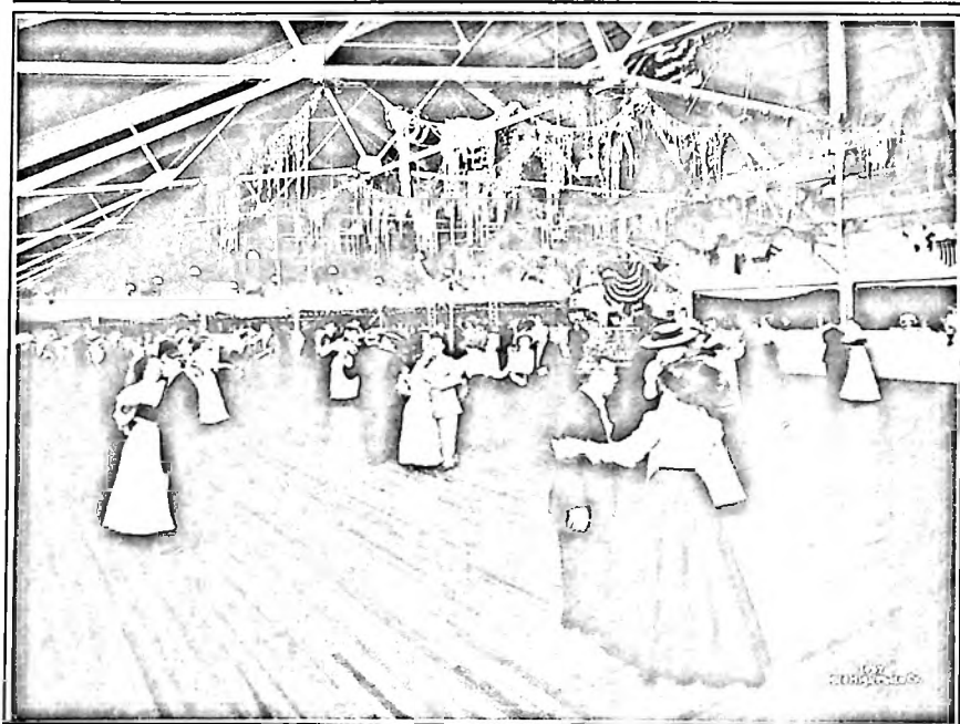
Inside the ballroom at Manhattan Beach
