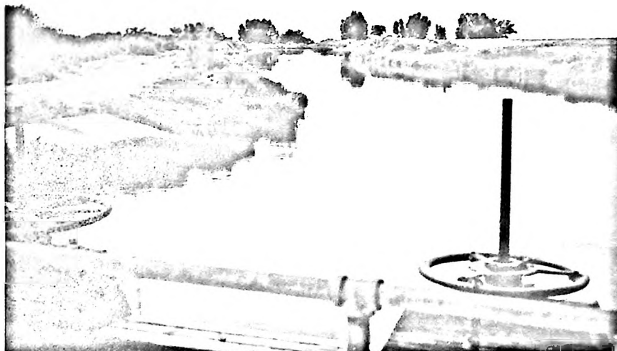
Outlet of the South Canal which delivers water from the Gunnison River via the Gunnison Tunnel to the Uncompahgre Irrigation Projects, between Montrose and Colona. Mel Griffiths photo.
