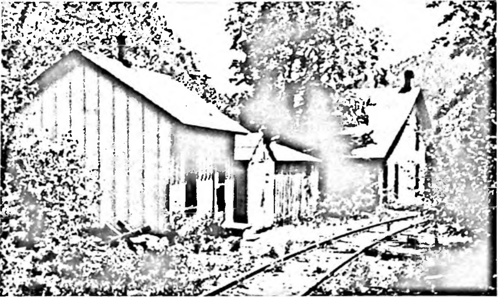
The weed-grown trackage at the Fall River sectionhouse shows the neglected maintenance of the right-of-way, especially the lack of track drainage.
