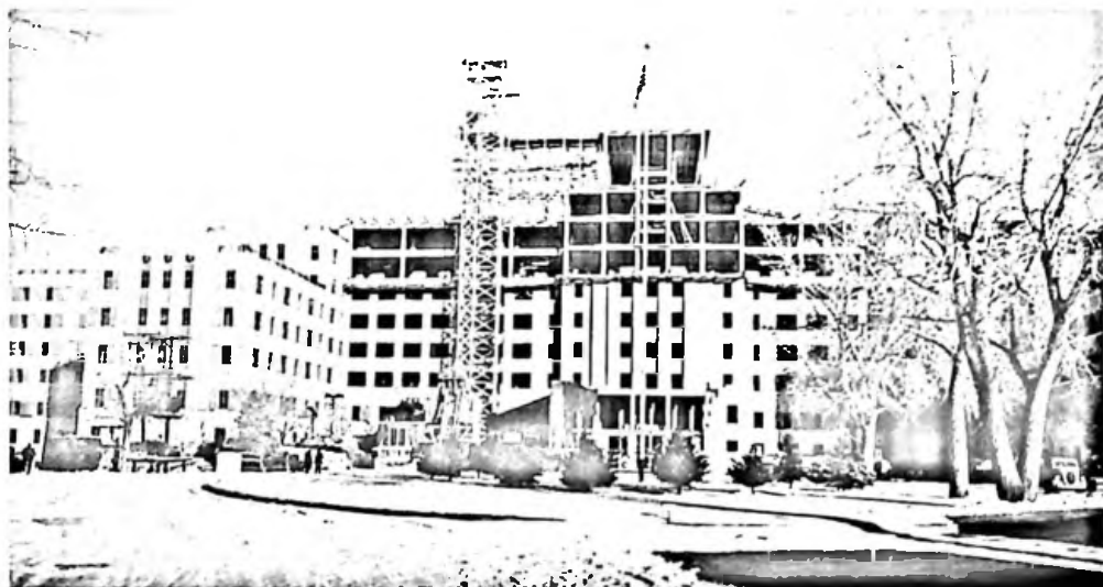
New hospital under construction, January 1940.
