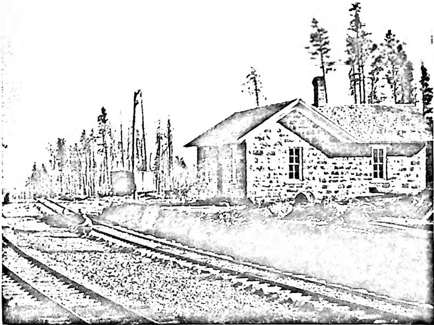
Station House, Summit of La Veta Pass, Late 1870's. (Hawkins Photograph.)
