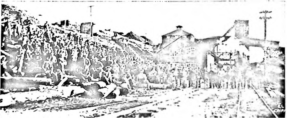
The El Paso Mine circa 1900. 200 men worked in stope at one time.
