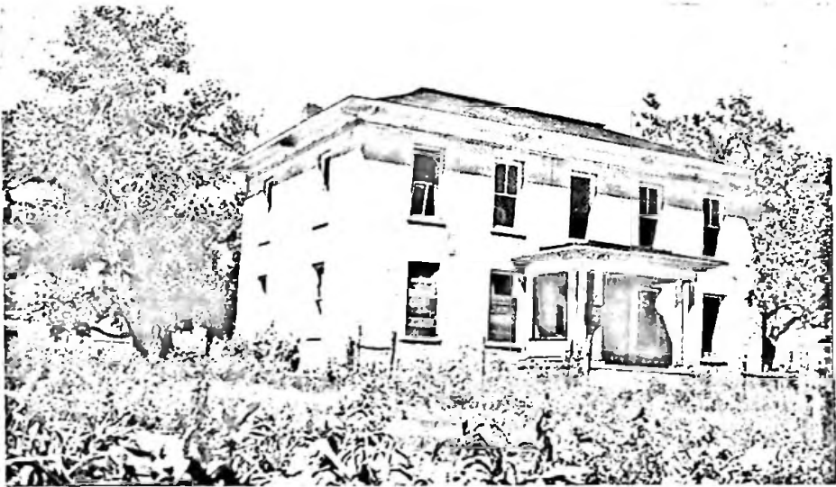
THE BRADFORD STAGE STATION IN 1954
